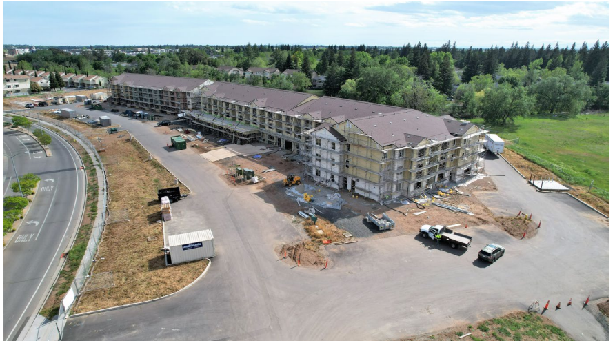
Photo courtesy of Sunseri Construction
